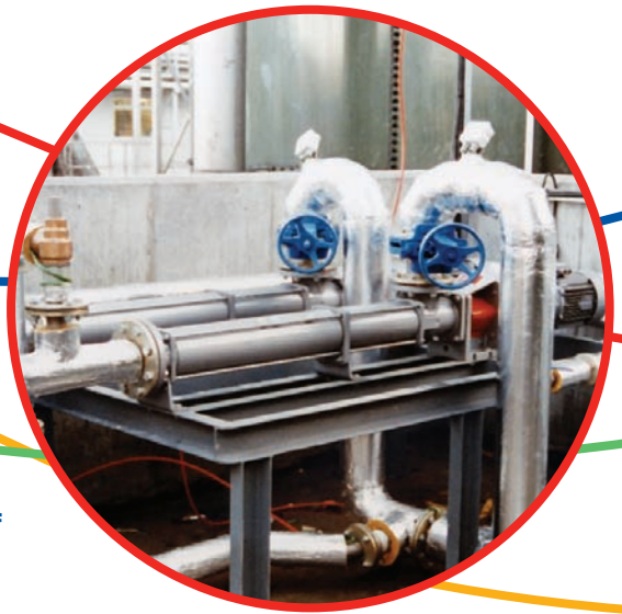
Pumping of slurry mix
